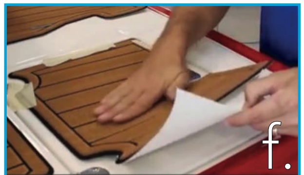
Apply downward pressure from the center working your way outward
